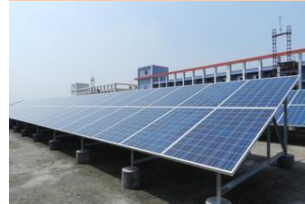
Concrete Roof System
