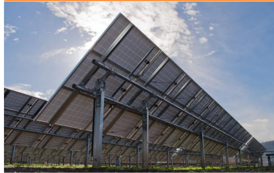
Single Axis Tracking System
