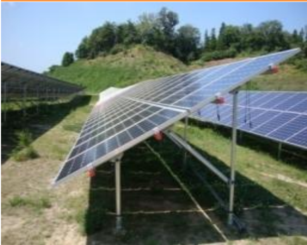
Ground Screw Foundation
